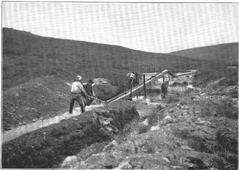
A. SLUICING ON HANNUM CREEK.
