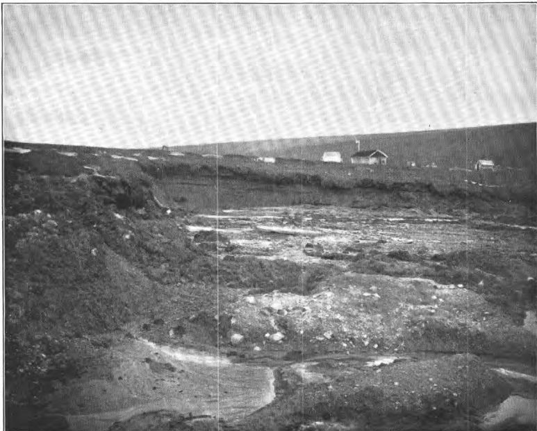
B. BENCH CLAIM ON CANDLE CREEK, SHOWING 12 FEET OF ICE ABOVE THE GRAVEL.
