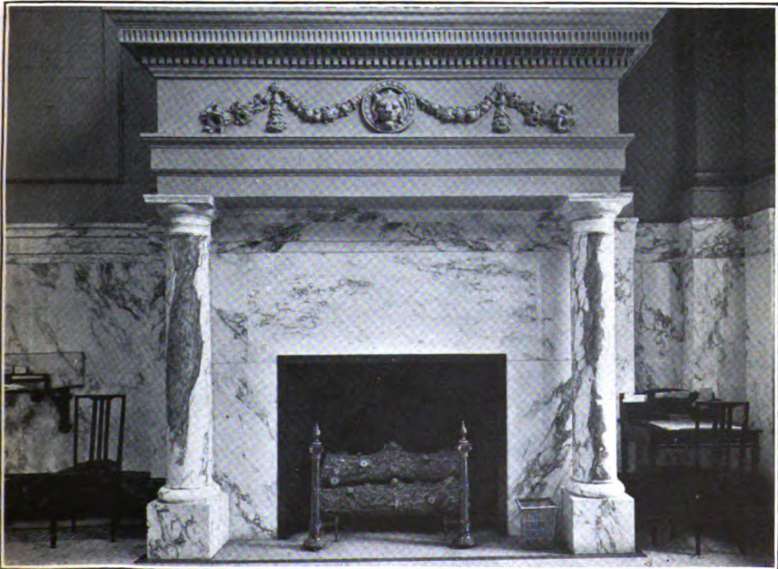
B. MANTEL AND WAINSCOTING IN FIRST NATIONAL BANK, HAZLETON, PA. Muscovitic calcite marble, "A. and S. Bonazzo," from West Rutland.
