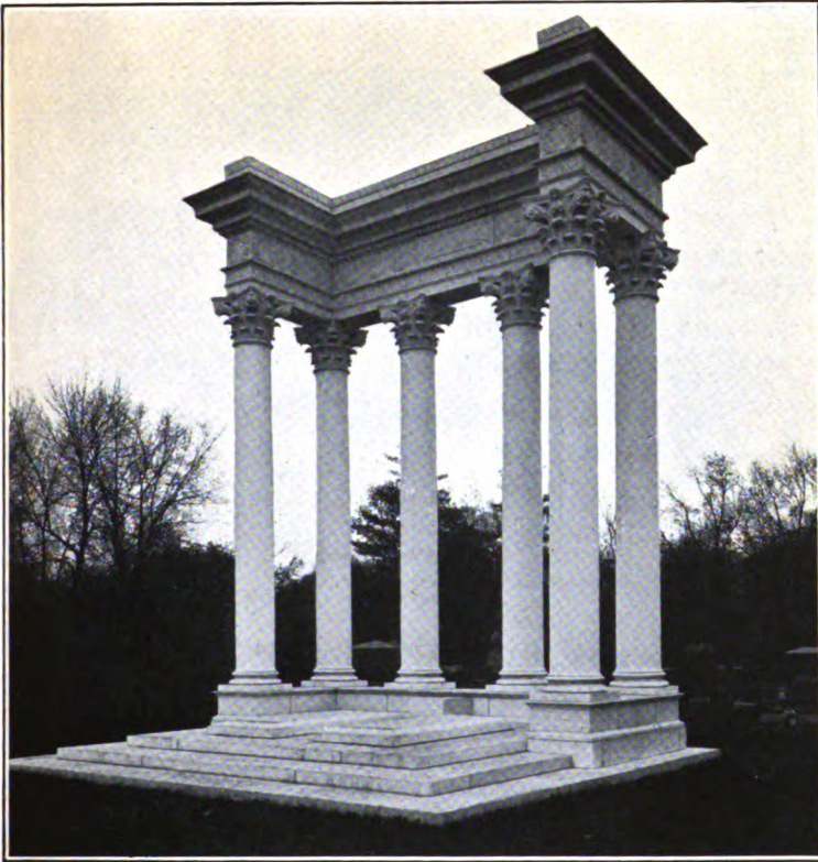
A. KIMBALL MONUMENT, GRACELAND CEMETERY, CHICAGO, ILL. Columns of "second statuary Rutland" calcite marble.
