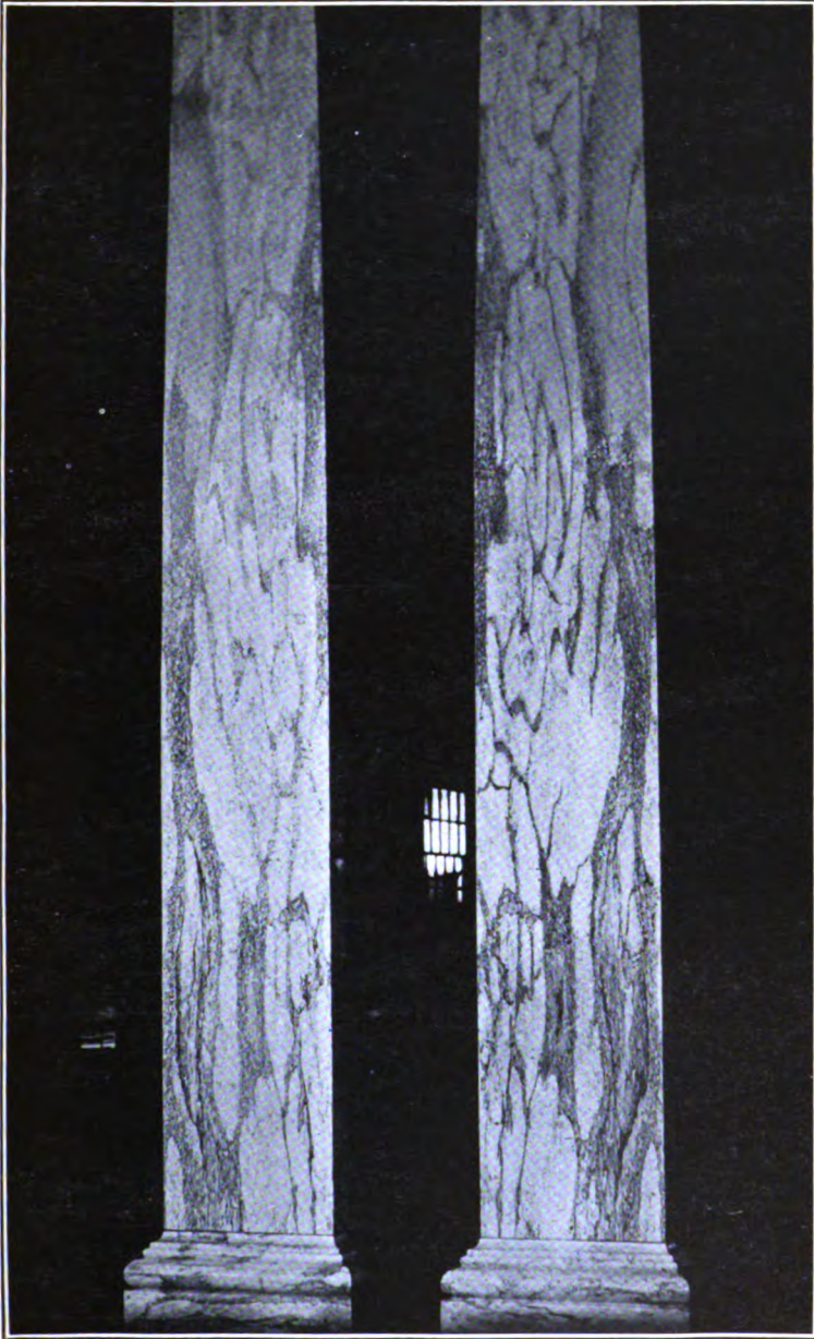
POLISHED PILASTERS OF ACTINOLITIC CALCITE MARBLE FROM "GREEN BED," VALLEY QUARRY, SOUTH DORSET.
