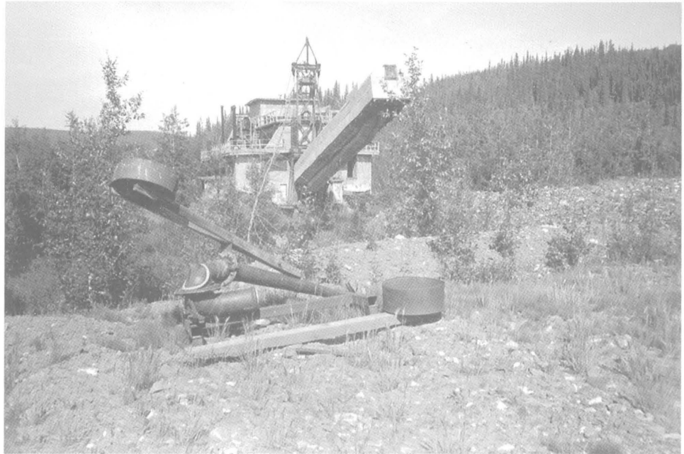
Figure 27 THE DREDGE IN CHICKEN CREEK (east-central Alaska), which operated between 1959 and 1967. Hydraulic monitors in foreground were used to mine creek and bench gravels here during the 1970's.
