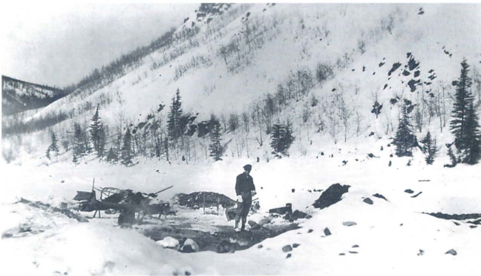
Figure 13 WINTER MINING IN BED OF FORTYMILE RIVER, 1921 at "Swansons Diggings" in east-central Alaska. The ice was picked away and the frozen gravel was thawed to bedrock using open wood fires. Photo courtesy of University of Alaska Archives, Fairbanks, Alaska.
