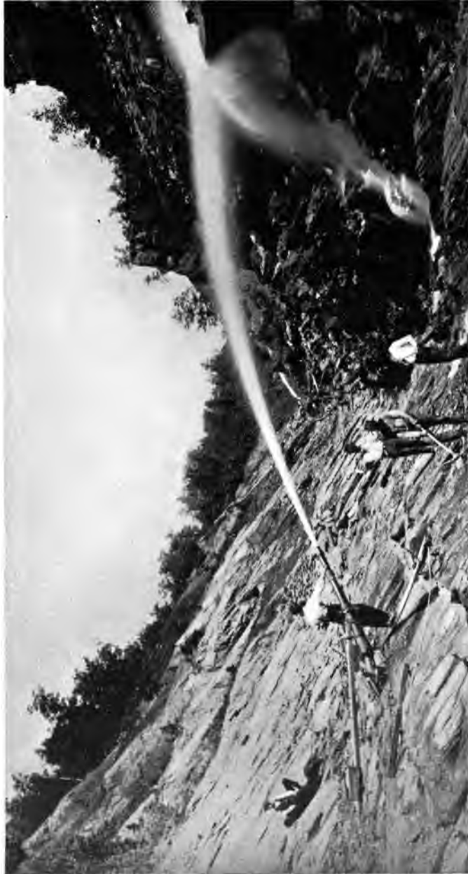
DAHLONGA METHOD OF MINING, SHOWING GIANT AND GROUND SLUICE.
