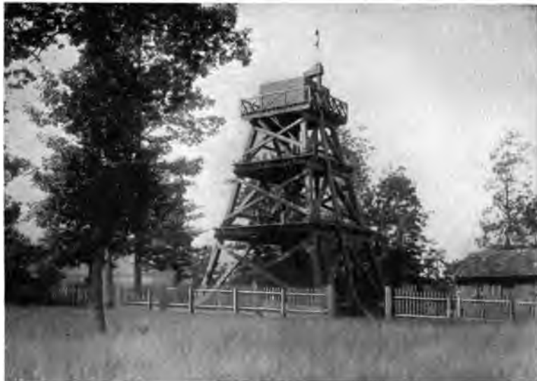
STAND-PIPE, PARKER MINE.
