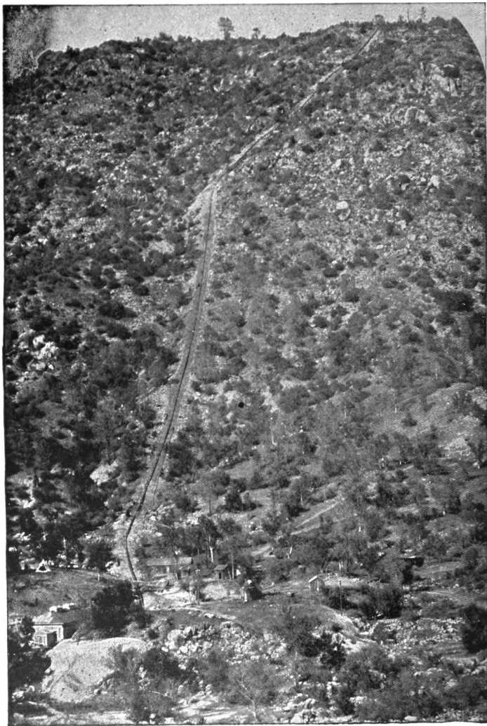
Fresno Power Plant.
