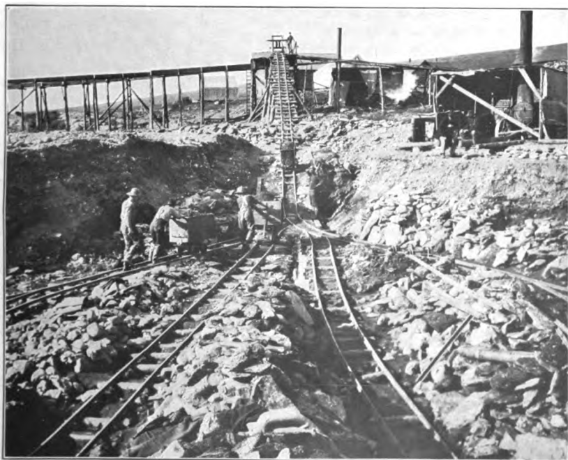
B. PLACER MINING WITH TRACK AND INCLINE ON OPHIR CREEK.
