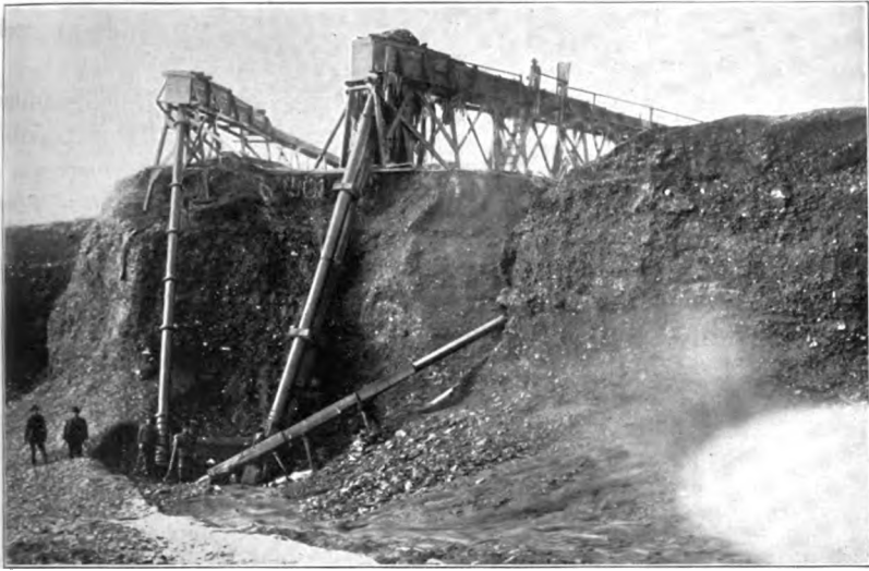
A. HYDRAULIC ELEVATOR ON GLACIER CREEK.
