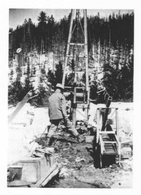
FIGURE 9. – Hillman 4-inch Airplane drill. This compact, skid-mounted machine is widely used for reconnaissance-type prospecting.
