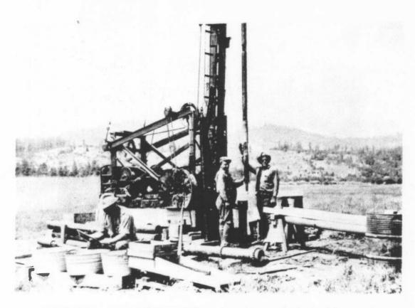
FIGURE 10. -A typical placer drilling set-up. Note rocker for washing samples.
