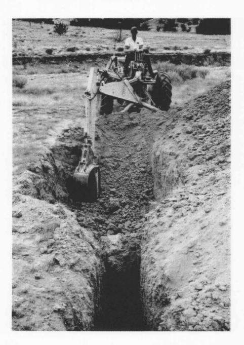
FIGURE 6. – Backhoe excavator digging trench in placer ground. Hand-dug channel samples were later taken from the trench walls.
